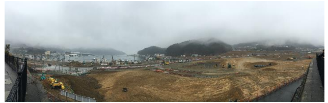
Figure 4 An unfamiliar townscape created by reconstruction in Onagawa Town.
