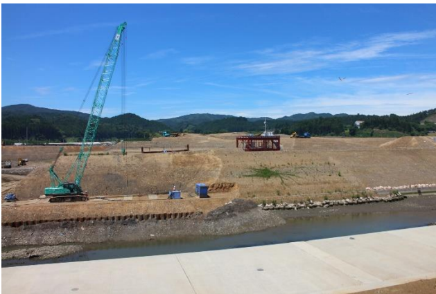
Figure 2 Cut and fill project in Minami Sanriku Town.
