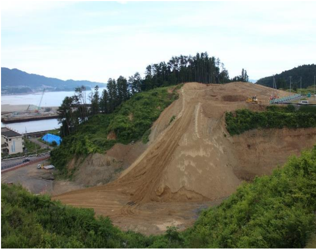
Figure 1 Cut and fill project in Rikuzentakata City.
