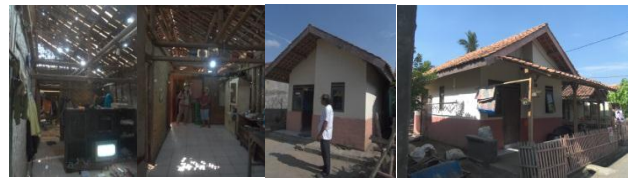
Figure 7 (a) & (b) Poor ventilation and opening considerations for the original dwellings; (c) & (d) Opening considerations for Habitat homes
